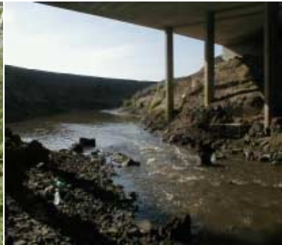
Figure 4.6. The Reclamation Ditch at Highway 183.
