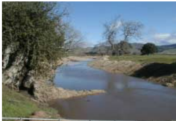
Figure 5.12. A small earth dam, minutes after breaching, made of sand above GAB-BOR. It is presumed that this was the reason for no flow at GAB-BOR during previous events.
