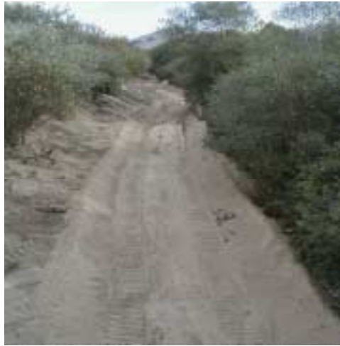
Figure 6.1. Bulldozing of the channel between GAB-HER and GAB-CRA in August of 2000.
