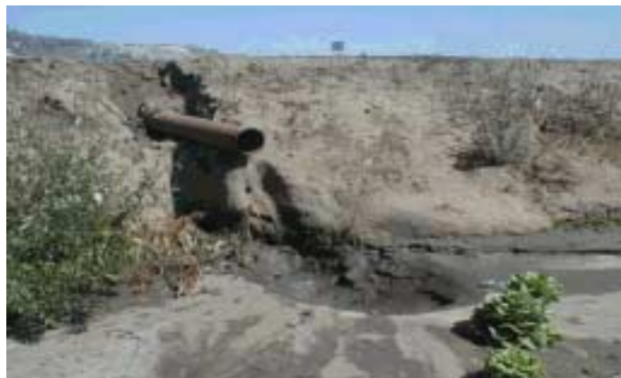
Figure 3.1. Agricultural drainage pipe feeding into Gabilan Creek. Note the difference in sediment color between just under the pipe (dark mud) and the remainder of the bed material (sands). Also note the lettuce growing in the lower right hand corner of the picture. The adjacent cropland here is a lettuce field.
