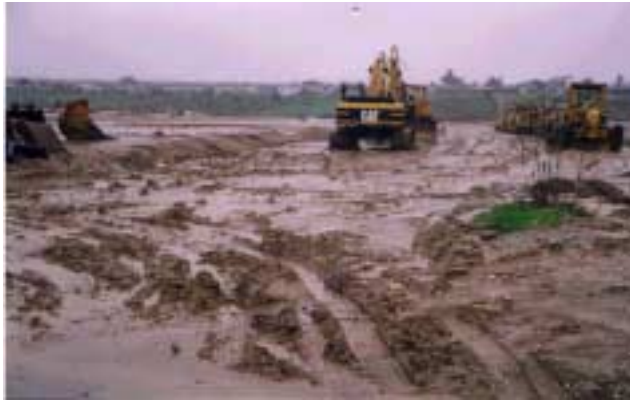
Figure 3.3. A construction site in Salinas near Gabilan Creek.
