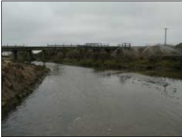
Figure 6-3. Location: Reach 1 Section 1, showing confluence with Tembladero Slough, incised channel, and lack of riparian vegetation (Photo: JulieHager)
