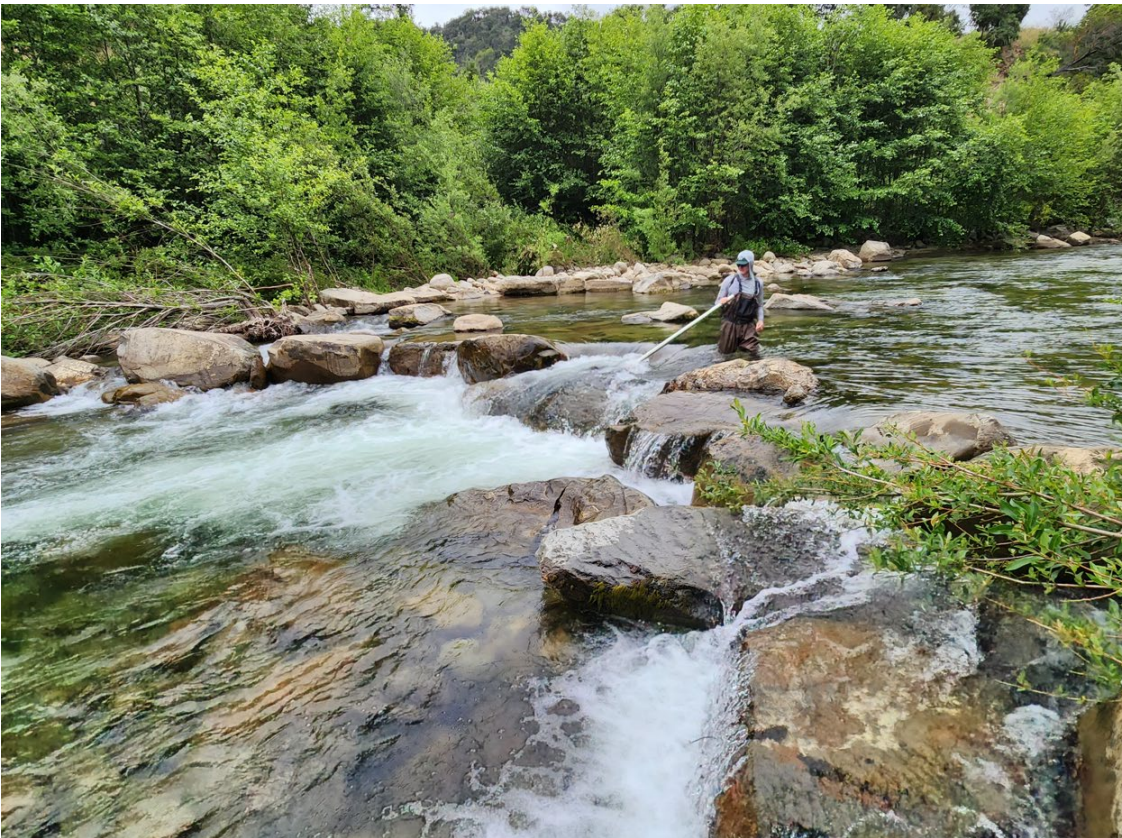
Figure 4. An original constructed arched rock weir (step-pool unit) with 70 cfs of flow. Fish can pass this feature with a modest jump from a 2.5 foot deep launching pool or by burst swimming up the center chute, which has >1 ft depth in a gap between rocks.
