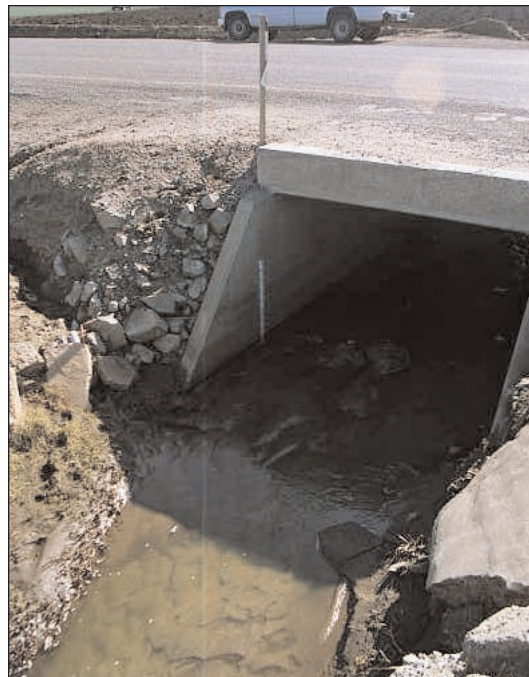
Figure 3.5 Site CHU-CRR: Downstream of River Road crossing; staff plate visible on right bank side of road crossing (photo: Fred Watson).
