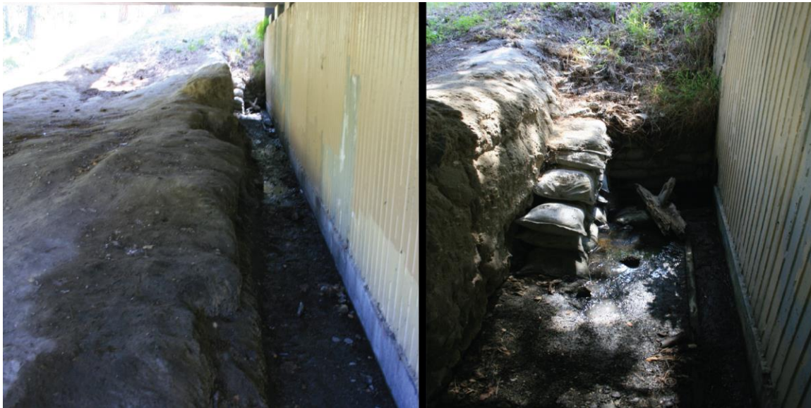
Figure 21: Drain diversion from Del Monte Center Bridge. To the left is the channelized path diverting water to the north, and the image on the right shows the sandbags used at south drain.
