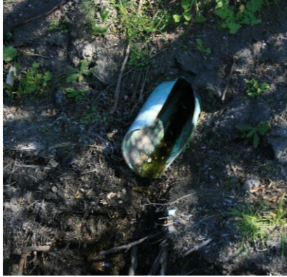
12-inch PVC pipe, near Whole Foods, located on the East Bank of upper Majors Creek
