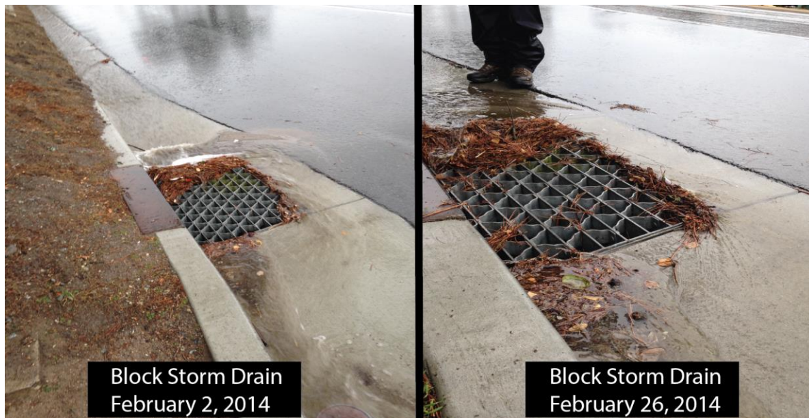
Figure 26: Storm drain at the SE corner of Munras Ave and El Dorado St. Drain was observed to become blocked with debris on several occasions and the blockage rerouted water around the drain and into the Majors Creek watershed.
