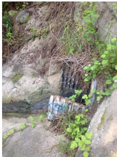
36-inch CMP culvert under Don Dahvee Lane, located in-stream to convey flow under road.
