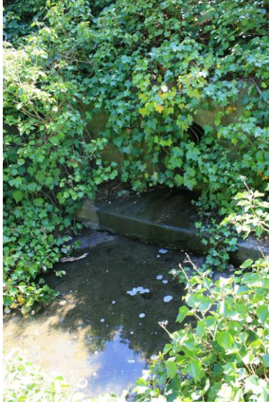
36-inch culvert under Del Monte Center entrance, located in-stream to convey flow under road.
