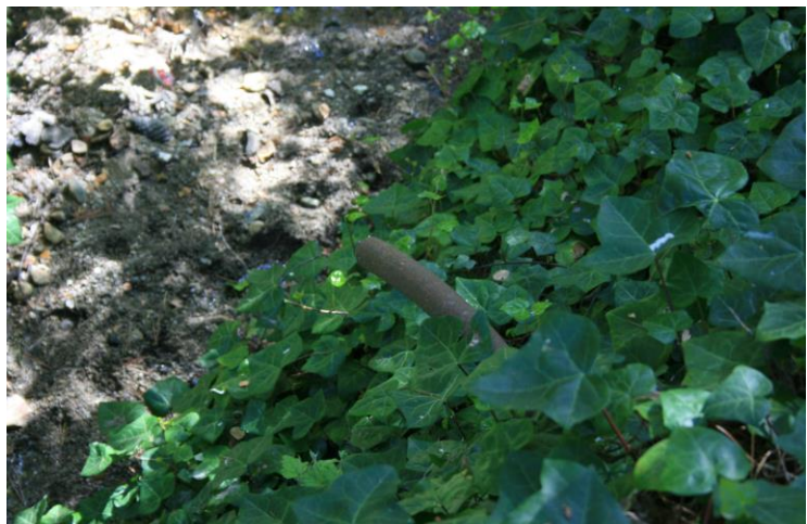
Figure 23: 1.5" metal pipe coming into Majors Creek.
