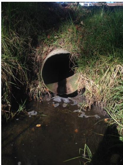
18-inch cement pipe, near Whole Foods, located on West Bank of upper Majors Creek
