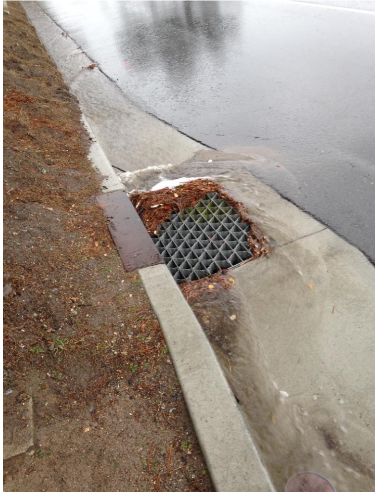
Figure 6: Storm drain at SE corner of Munras and El Dorado intersection blocked with debris during Feb 28 th rain event. Runoff was rerouted past the drain, down El Dorado Street, and into the storm drain that feeds into the MC01 culvert.
