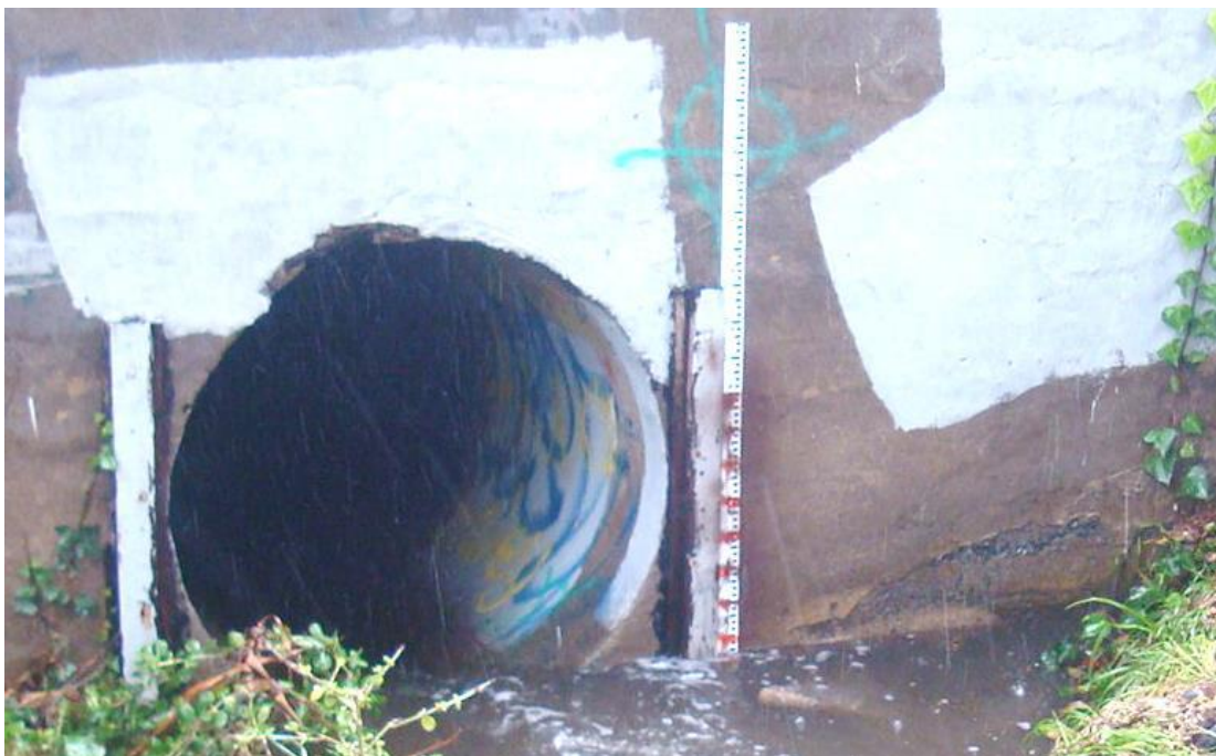
Staff plate installed at lower end of Greenwood Park (plates are visible to right of culvert entrance)
