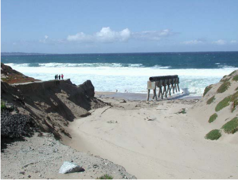
Figure B8: Storm drain outfall on Former Fort Ord compromised by coastal retreat. Canyon is formed by rapid undercutting and vertical failing of buried storm drain pipe (see Fig. B9). Photo by David Norris September 2002. See Figure 18 for map view of the eroded canyon.
