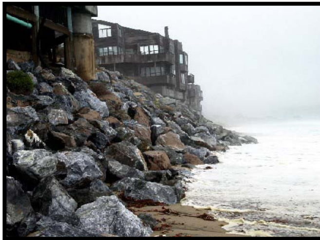
Figure 7: Sea wall protecting Ocean Harbor House Condominiums. December 9, 2004.
