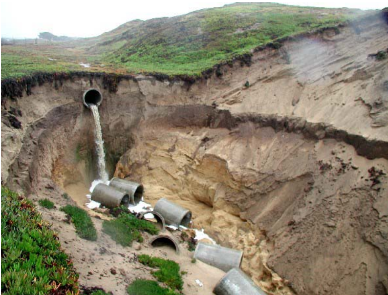
Figure B9: Storm drain outfall on Former Fort Ord compromised by coastal retreat. Waterfall undercuts weak sandstone substrate causing subsequent collapse of storm drain pipe sections. (see Fig. B9 for original location of outfall). Photo by David Norris September 2002. See Figure 18 for map view of the eroded canyon.
