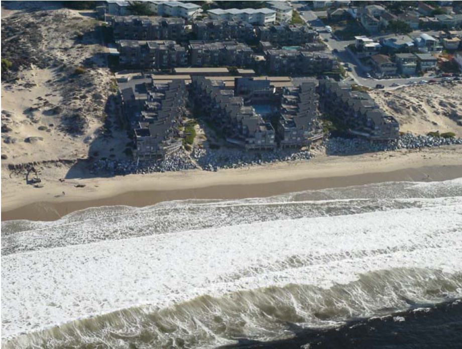
Figure B4: Ocean Harbor House Condominiums on October 31, 2004 showing site after large rock was placed to create a sea wall.
