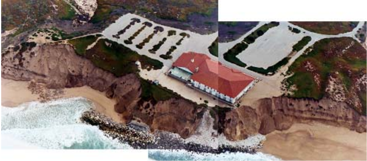
Figure B1: Stillwell Hall in 2003 showing sea wall compromised by unrestricted retreat of adjacent sea cliffs. This photo illustrates the “peninsula effect” produced by local hardening of a retreating coastline. Note sand cones and sand aprons transferring large volume of sand from sea cliff to beach.
