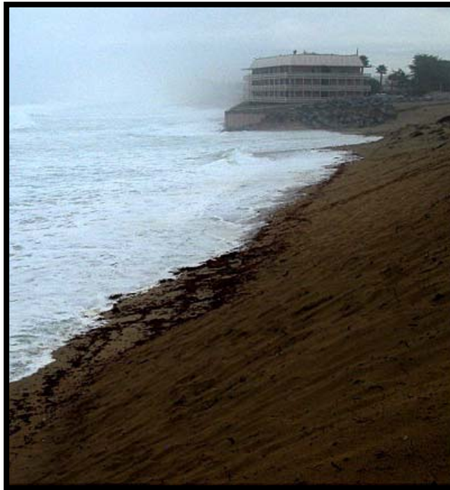
Figure 26: Peninsula effect present at Monterey Beach Resort at very high tides (5.98 ft) and high swells (15.5 ft; 16 second period) of December 9, 2004. Note large rock placed along wall damaged by high seas in December 2002 (Smith, 2005). There is normally a broad beach in front of the Resort, during lower surf and normal tides.
