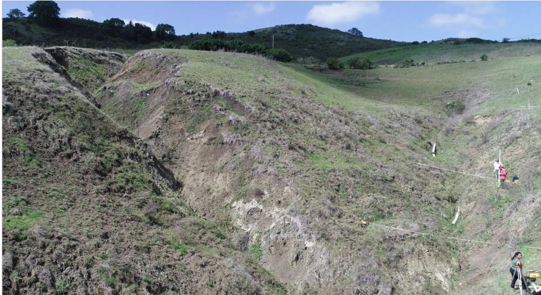
Figure 26. Gullies related to culvert drainage erosion. Right gully with surveyors terminates at the culvert labeled “2” in Figure 22. Broken white culvert pipe visible in thalweg is also visible in Figure 24. Left gully is feature number four in Figure 22, also shown in Figures 24 and 25. Image from Smith et al. (2016).
