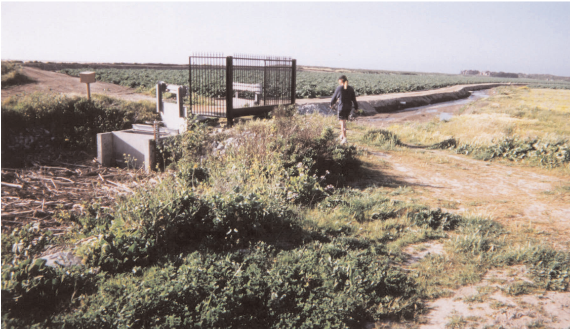
Figure 2.9 The Old Salinas River Channel and flow gates. This channel still occupies the historical route of the Salinas River from the lagoon northward to Moss Landing Harbor via the Potrero Road Tide gates.
