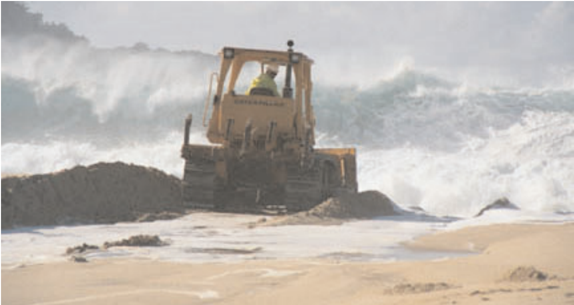
Figure 4.1 Monterey County Public Works bulldozer in the process of breaching the Carmel Lagoon during the afternoon of December 3, 2001.
