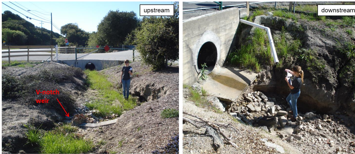
Figure 7 Upstream aggradation and downstream incision in the Arroyo del Rey channel at the Laguna Seca Raceway entrance.
