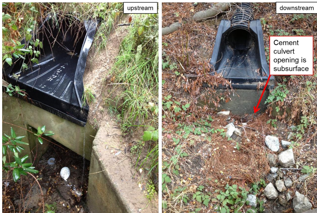
Figure 22 Square, concrete culverts connect the South Boundary basin to Frog Pond. The culvert is filled with sediment at the downstream end. The black, circular culverts drain runoff from General Jim Moore Blvd.
