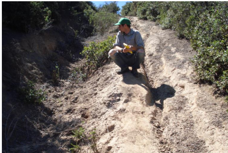
Figure 20 Erosion on an old army road within the South Boundary basin.
