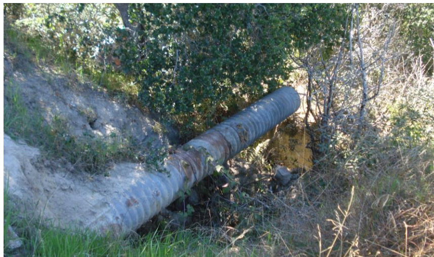
Figure 21 Outfall pipe extending from beneath South Boundary Road into the South Boundary basin. A deep ravine has formed beneath the pipe.
