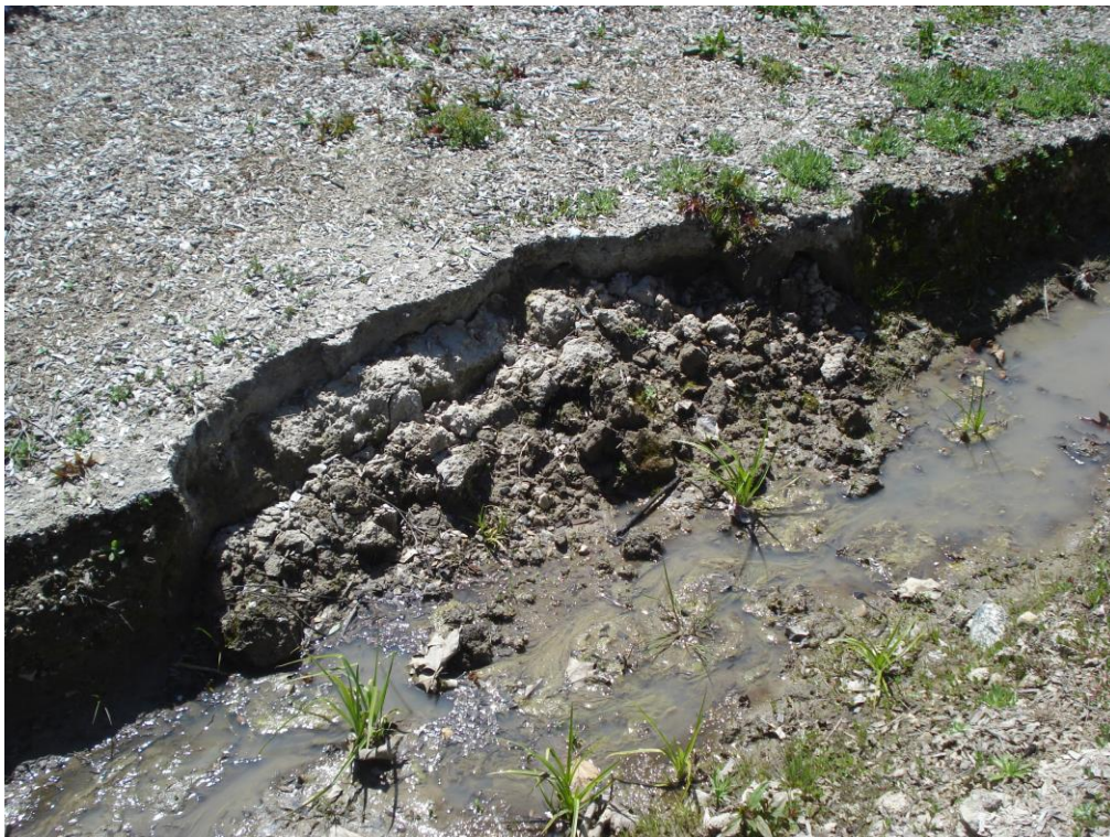
Figure 6 Erosion of channel edges near Laguna Seca.
