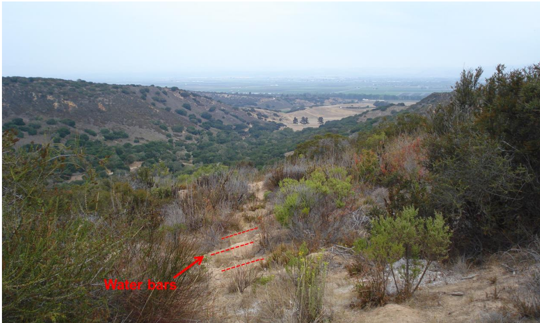
Figure 25 Water bars are created to allow for runoff accumulation near the roots of plants (Photo taken on BLM land in former Fort Ord).
