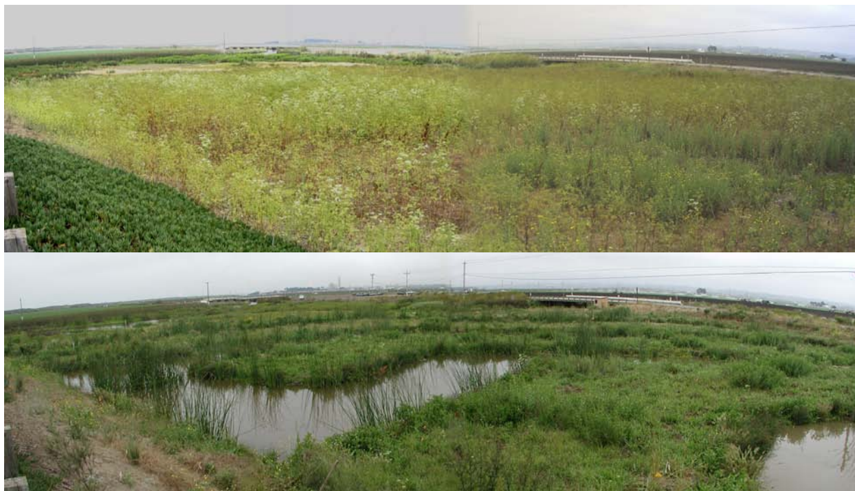
Figure 12.3. The upper photo is Pt 2 before construction taken 7/7/05. The site was dominated by weeds and ponded water did not collect in this upper portion. The lower photo is Pt 2 after construction on 7/11/06. In addition to all of the work that went into the main wetland area, Iceplant was also removed from alongside the road and replaced with natives (lower left corner of photos).
