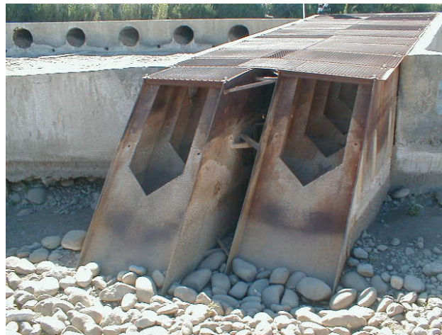
Figure 11.2 The Thorne Road crossing and fish ladder on the Arroyo Seco River. (Photo: Joel Casagrande, 29 Sep. 2001)
