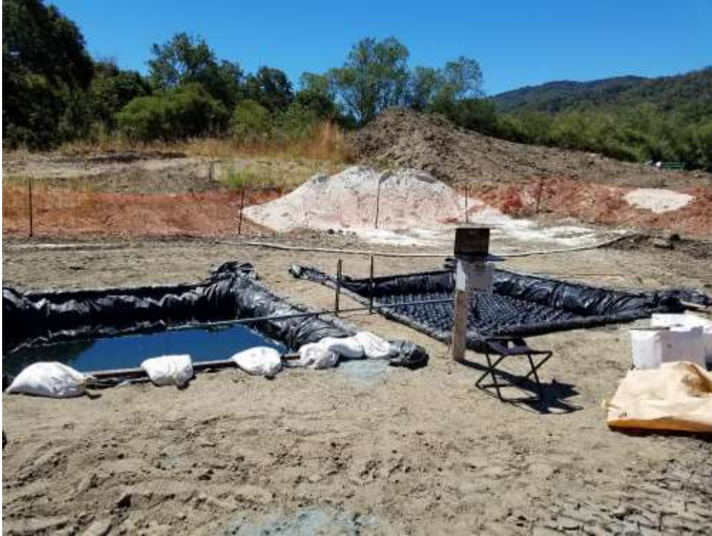
Figure 3: Two evaporation ponds. Left pond is open, and the right pond is covered with plastic floats.
