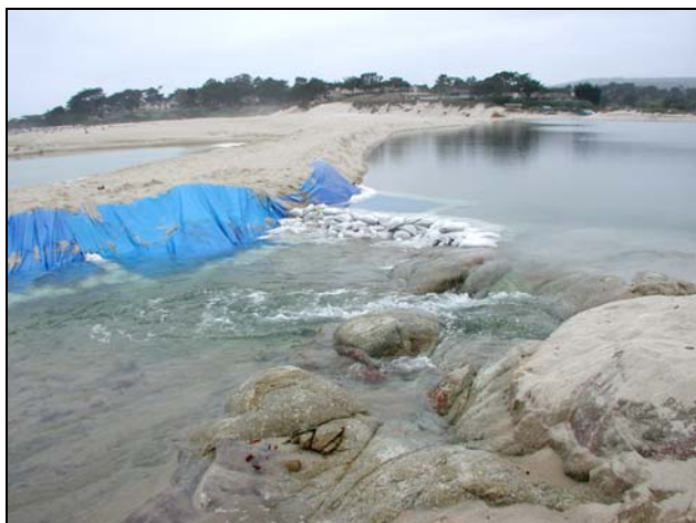
(c) The flow of the river out to the ocean was confined to the rock sill at the southern edge of the main lagoon with tarps and sandbags (19 Jun 2006).
