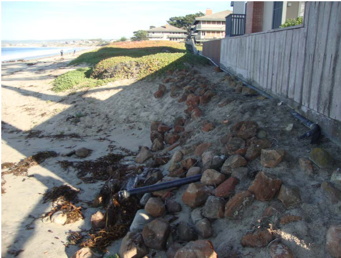
Figure 3. The northwest corner of Del Monte Townhomes. Small riprap was placed to protect a fence and drain pipe. Photo was taken November 11, 2012, shortly before the nourishment project began.
