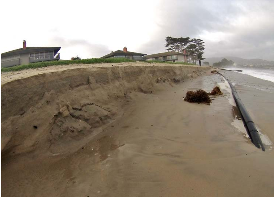
Figure 11. Significant berm erosion, indicated by tall erosional scarp, occurred during the king tide of 12/21/2014. The extent of erosion is indicated by the exposed black dredge slurry pipe, which had been buried under the berm.
