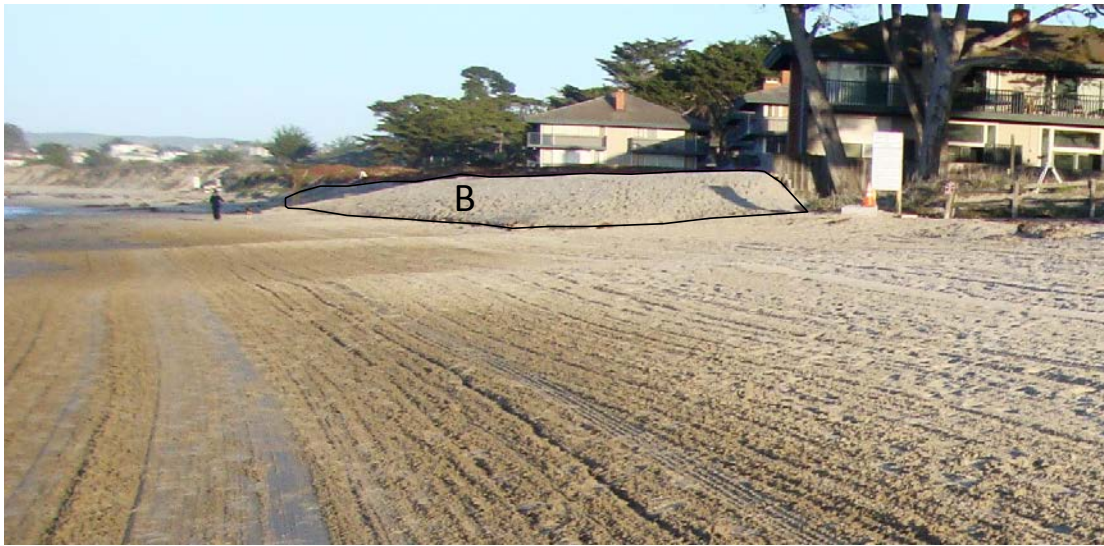
Figure 5. The nourishment berm (B) is shown very soon after completion of the first nourishment event in the winter of 2012/2013. View is eastward, toward the fence shown in Figure 3.
