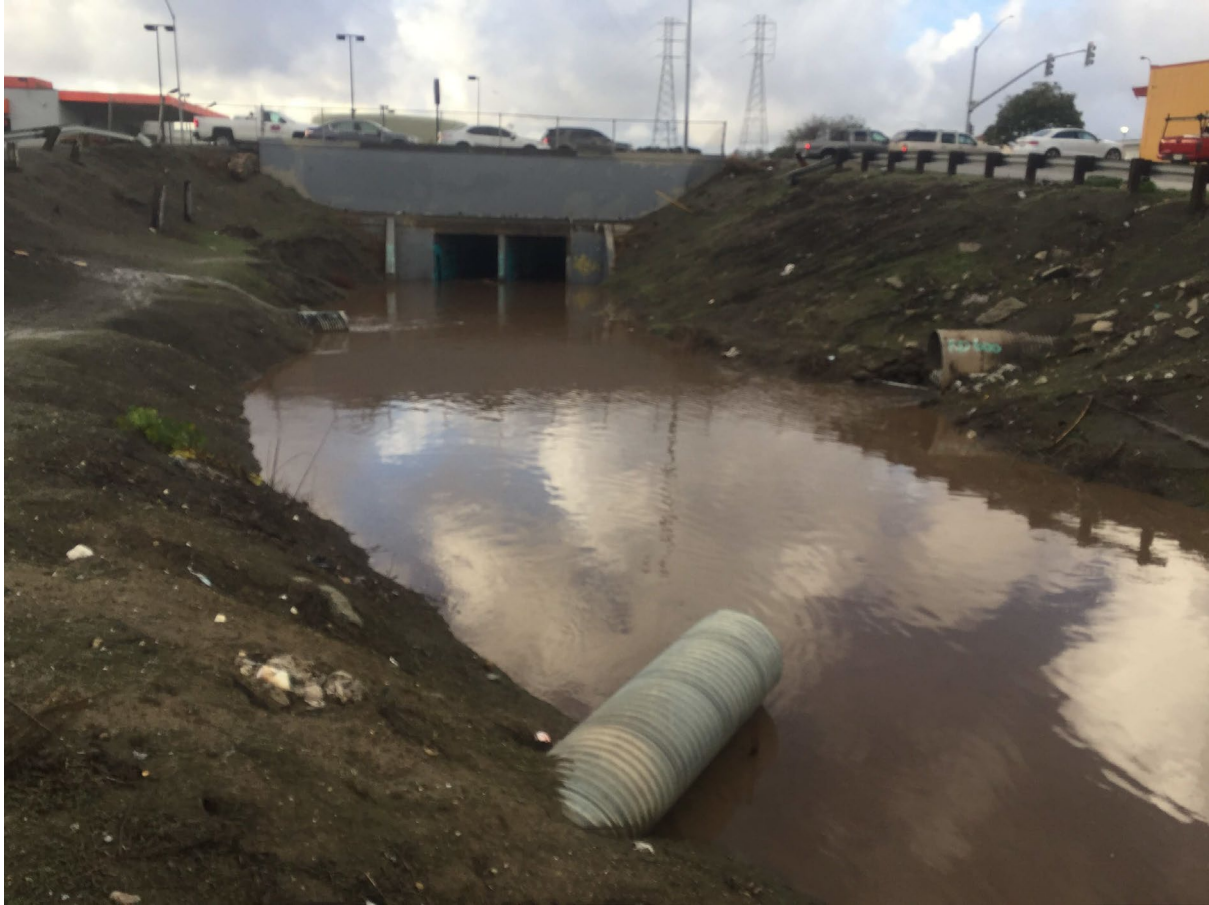
Figure 7. North Main Street culverts on November 29, 2018 after heavy rain. The small 36-inch culvert is under water.
