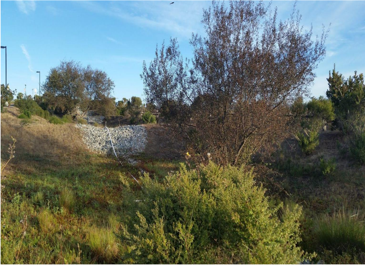
Figure 4-2: An example of a bioswale configuration that could be implemented at POM. This bioswale is adjacent to Pajaro Valley High School .
