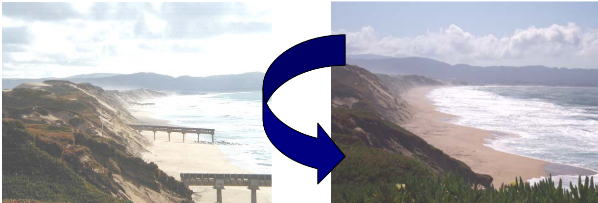
Storm drainage outfall removal – Before and After
